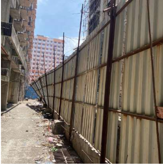
Temporary GI Boundry wall
