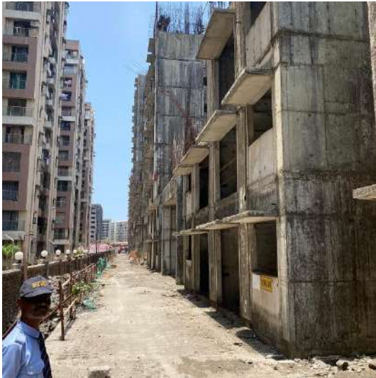
9 Mt internal Road
