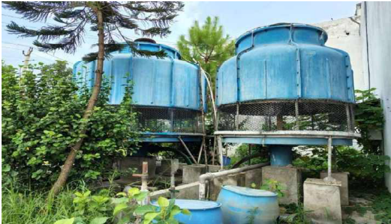
FRP COOLING TOWER NEAR GATE CONNECTED TO CHILLER SYSTEM
