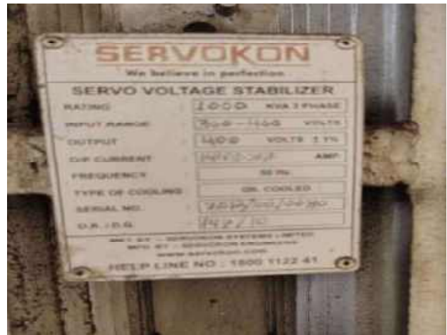
MAINS POWER CAPACITOR BANK AND PCC PANEL WITH SERVO VOLTAGE STABILISER TRANSFORMER NAME PLATE
