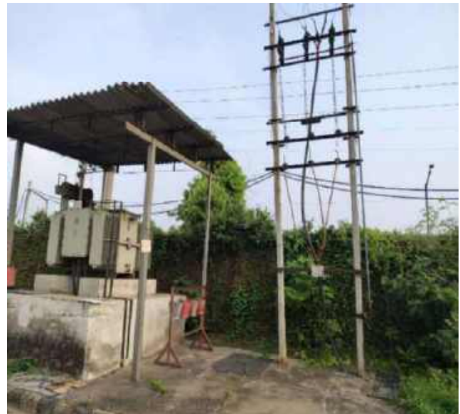
STATE ELECTRIC SUPPLY POINT/ SHED - CEMENT POLE INTAKE STRUCTURE WITH AB SWITCH AND FUSE UNIT-2 NO.
