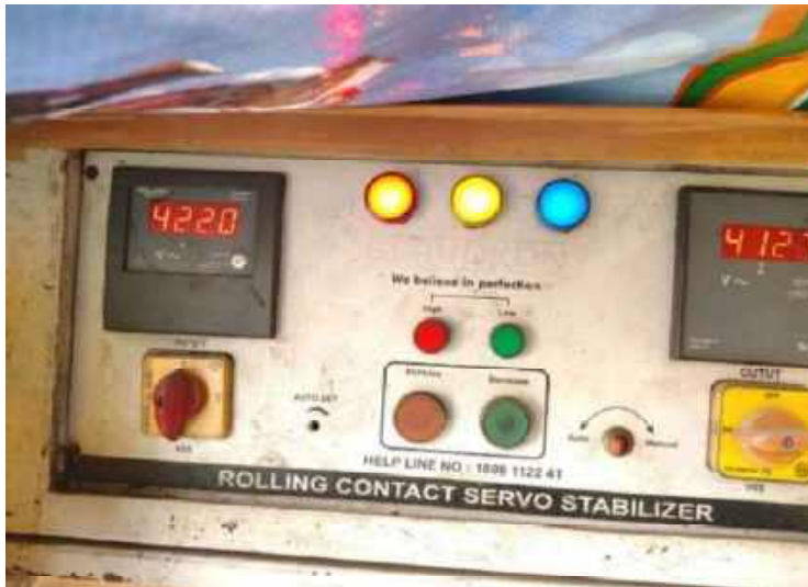
CONTROL PANEL FOR SERVO VOLTAGE STABILIZER
