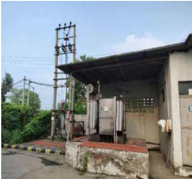
STATE ELECTRIC SUPPLY POINT/ SHED - CEMENT POLE INTAKE STRUCTURE WITH AB SWITCH AND FUSE UNIT-2 NO.
